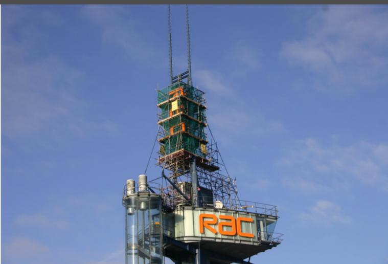
Hercules scaffolding was appointed by the RAC to provide high level scaffolding access platforms reaching some 120m in Height on the iconic RAC head office building overlooking the M5 / M4 interchange in Bristol.
