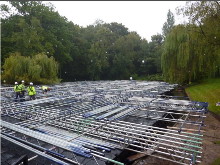
Hercules Scaffolding was appointed scaffolding contractor to Design and Install one of the largest floating scaffold stages ever created in the UK. The project involved designing and installing a scaffold stage and ballroom floor over a lake in Hampstead Heath London.
